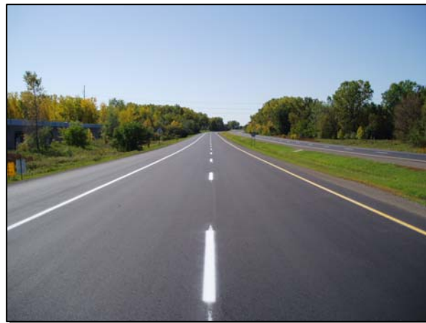
Figure 2. Ramsey CSAH 88 Completed.
