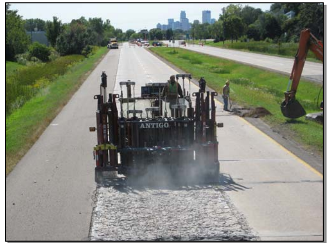
Figure 1. Rubblizing Ramsey CSAH 88.
