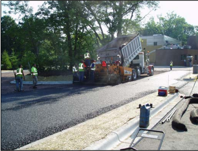
Photos 2 & 3. Porous HMA Pavement at the Unitarian Church in Mahtomedi, MN.
