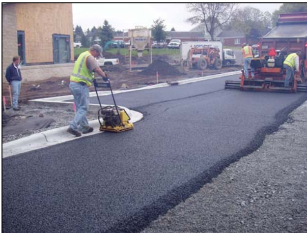
Photo 1. Porous HMA Pavement at the Ramsey Ramsey-Washington Metro Watershed District office building in Little Canada, MN.
