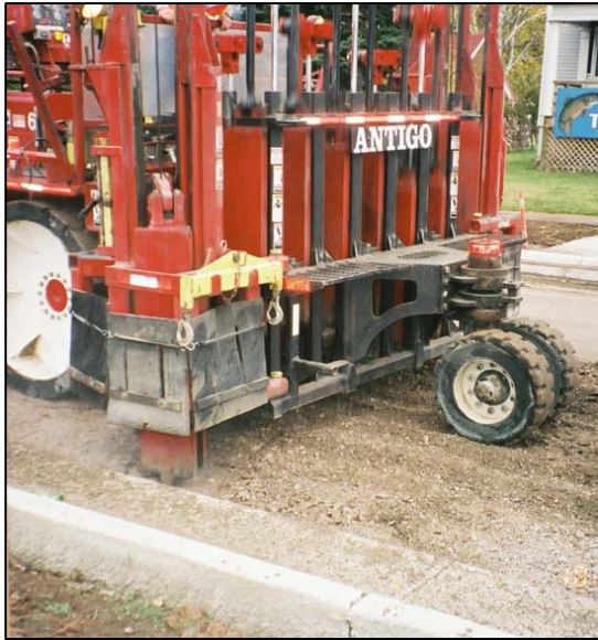
Figure 4 – Rubblizing adjacent to curb & gutter.
